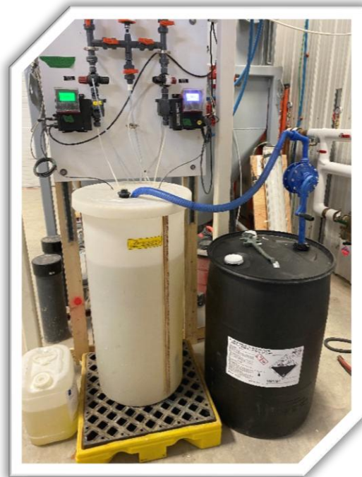
Figure 5: Chlorine Dosing
