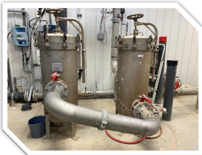
Figure 6: Cartridge Filters #2 & #1
