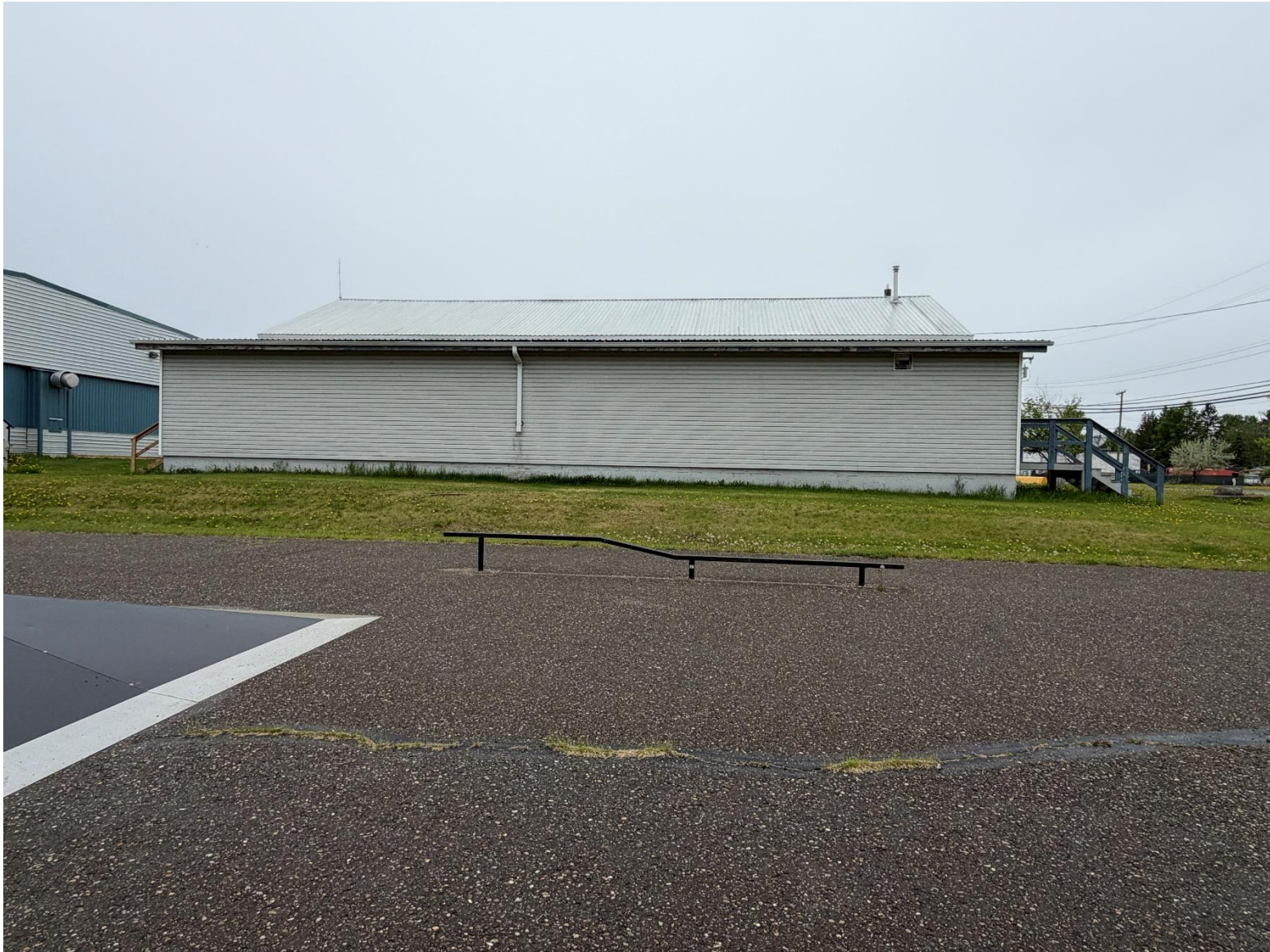
Photo 2: North Elevation, from Skateboard Park
