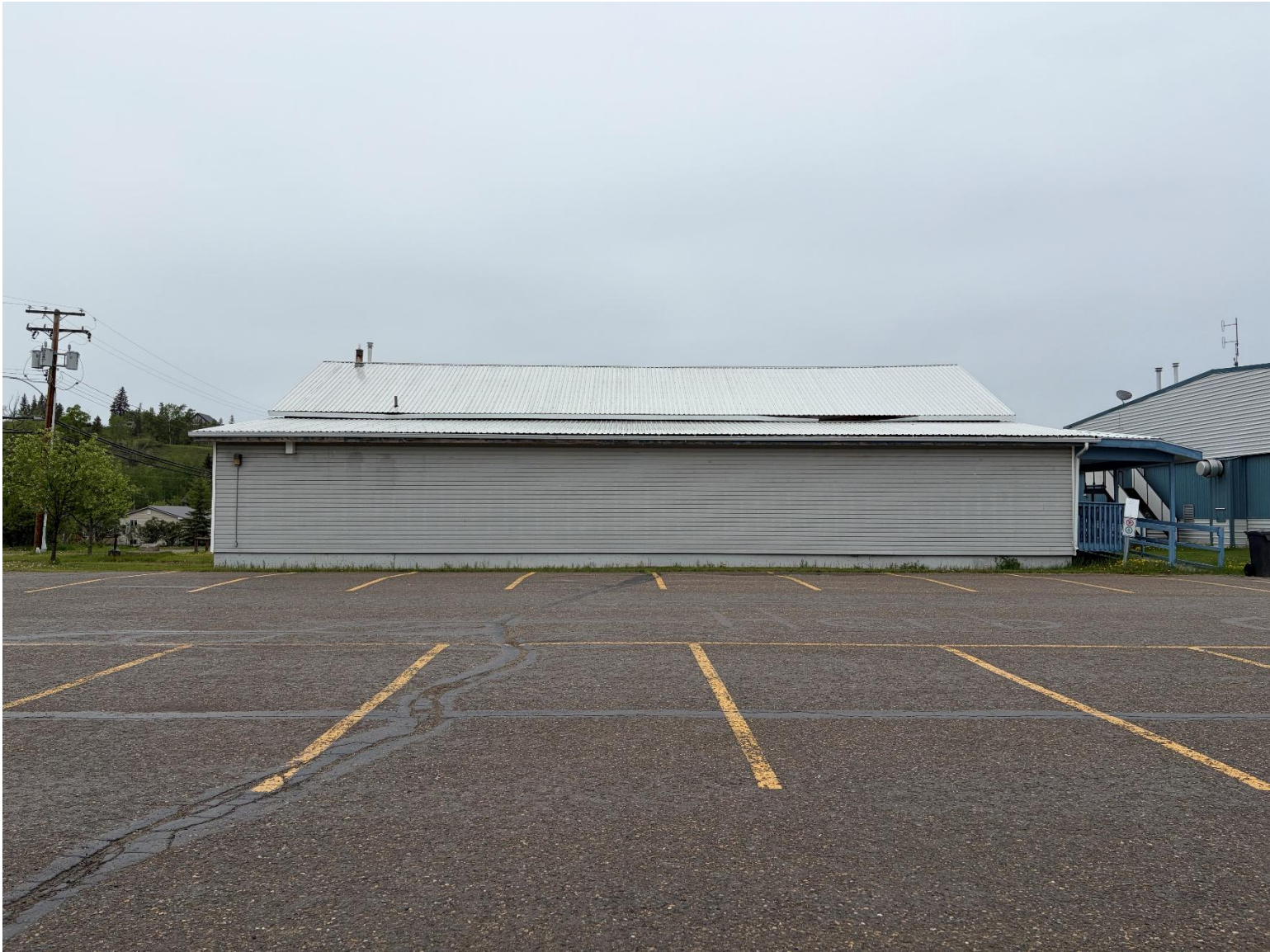
Photo 3: South Elevation, from Parking Lot
