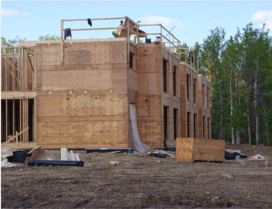
New 36 unit apartment building under construction on Paquette Ave. (August 2012)
