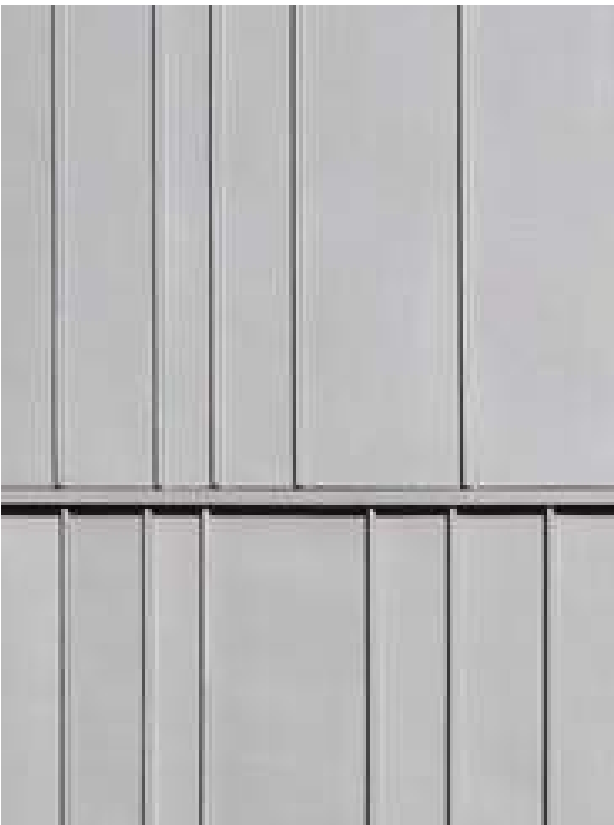
METAL CLADDING Corrugated sheet metal cladding
