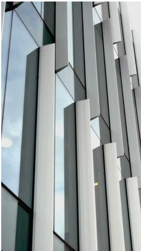
CURTAIN WALL GLAZING + FINS Clear Anodized Aluminum Double or Triple Glazed to be confirmed by Energy Modelling team
