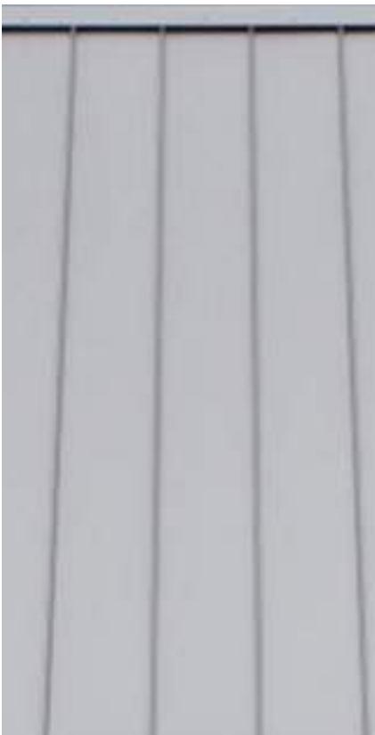
ROOFING Standing Seam Metal Roofing
