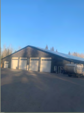
PUBLIC WORKS WITH A SOLAR ROOF LARGE FOOTPRINT
